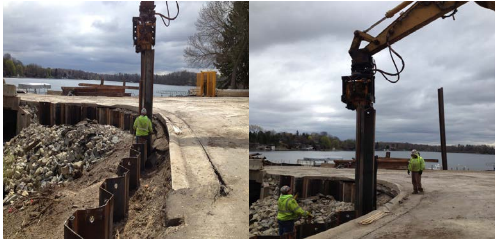
Sheet pile driving at Marsh Rd and CTH J
