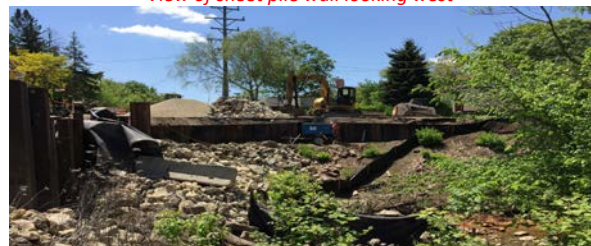
View of sheet pile wall looking west
