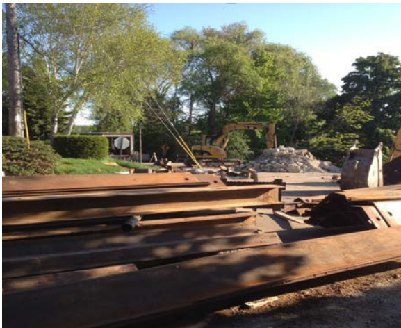
Construction Staging Area at CTH J & Marsh Road Intersection
