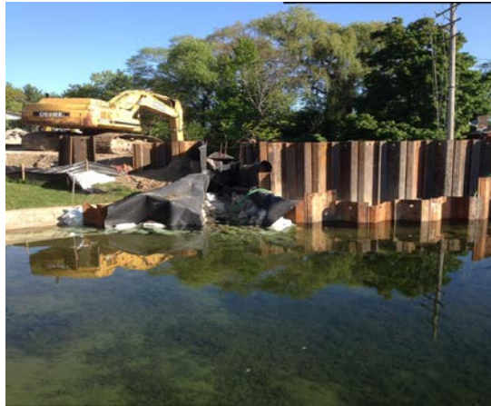
View of diversion channel & coffer dam looking north
