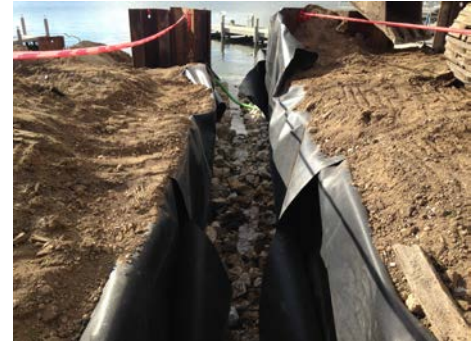
View of diversion channel looking south
